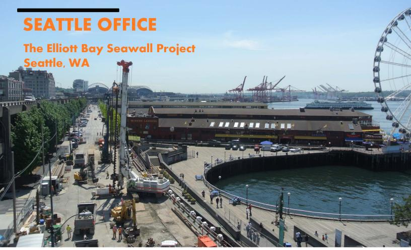
The Seattle Seawall was originally constructed between the years of 1916 and 1934 utilizing and estimated 20,000 old growth timbers that have been slowly eaten away from father time and gribbles (tiny marine borers that have an appetite for wood). Seattle's Seawall supports SR 99, Alaska Way, the ferry terminal, as well as major utilities. Seismic concerns are also an issue since everything behind the seawall from Alaskan Way to Western Avenue is built on top of fill.
