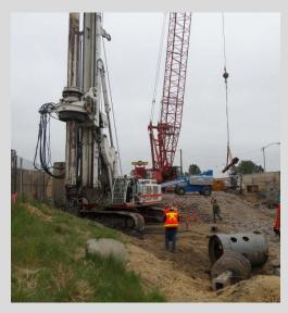
On April 8<sup>th</sup>, CJA began work on the I-205 @ NE Airport Way project in Portland, Oregon. The project for Hamilton Construction consists of four each 4-foot diameter bridge shafts up to 140-feet deep, a 4-foot diameter secant pile wall with 21 primaries and 23 secondaries, and five drilled shafts for sign poles. All shafts will be temporarily cased to tip using the SR-100 and 1.2-meter oscillator.
