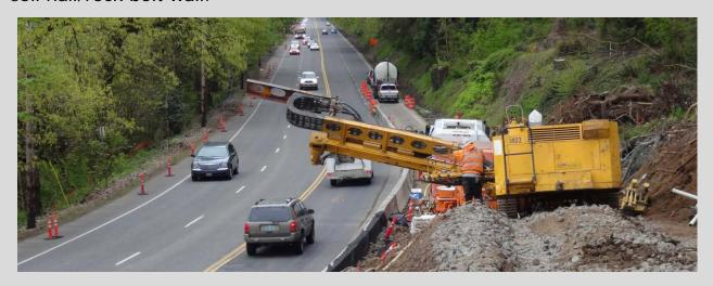
The AF-25 and Soilmec 312 will be used to install the soldier piles. Tiebacks, soil nails, and rock bolts will be installed using the Klemm 806, Reach-Over Rig, and Comacchio MC 602.
