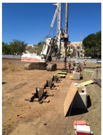
CJA was contracted by Clark/McCarthy to install OSHPD shoring for a new \$1 Billion hospital and design-build an adjacent parking structure in Palo Alto. Soldier piles, tiebacks, lagging, and internal bracing will be constructed for the below grade levels. CJA began in early April and the project is expected to take 9 months to complete.
