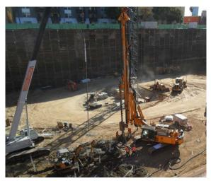
CJA is currently installing 47,000 square feet of design build soldier pile tieback shoring and 481 each tiedown anchors. Shoring was installed just east of San Diego's Petco Park and historic Gaslamp Quarter. This project is ongoing as of May, 2013.
