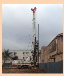
CJA was hired as a design-build shoring subcontractor for a multi-level mixed use retail and residential building in Huntington Beach, CA. CJA is installing 15,500 square feet of cantilevered soldier pile and timber lagging temporary shoring. Due to the dry, granular and sandy characteristics of the soil CJA elected to auger cast the toes and set the beams with the ABI.
