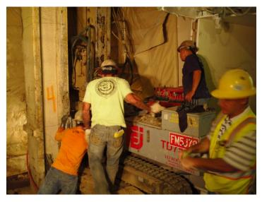
CJA installed 76 each difficult access micropiles with ultimate load capacities of 616 kips in compression and 313 kips in tension. During micropile installation Sharp Memorial Hospital was required to remain in full operation. The project was completed May, 2013.
