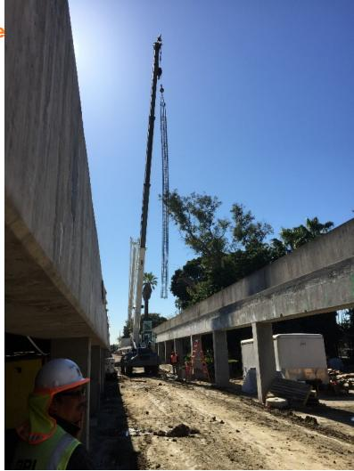
tasks. The reinforcing cages for the corridor piles had to be staged and secured on top of the parking structure's second level deck for the entire length of the corridor. Adding to the challenge was the groundwater that was encountered in all of the shafts. The standard CIDH piles were installed with a Geax DTC50 and the low overhead piles were installed with a Tescar 2.5. The micropiles were installed with a modified Klemm 803 using sections of continuous flight auger.
