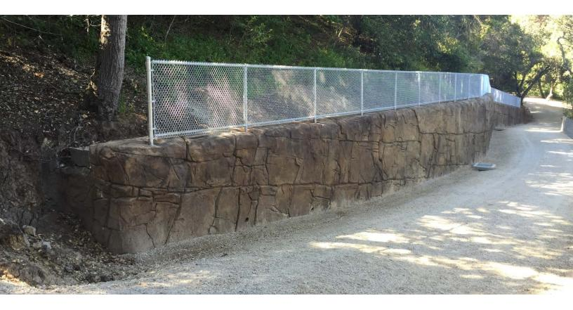
Redwood City contracted with CJA for the construction of a 2,580-square foot sculpted shotcrete retaining wall. In addition to the wall, the project consisted of various site improvements, including road work, installation of a gutter, and general drainage improvements. The purpose of the project was to prevent the existing slope from further erosion while widening the road.
