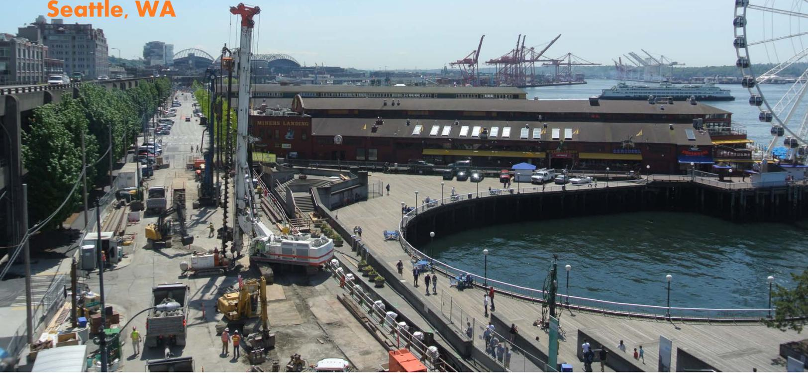
The Seattle Seawall was originally constructed between the years of 1916 and 1934 utilizing and estimated 20,000 old growth timbers that have been slowly eaten away from father time and gribbles (tiny marine borers that have an appetite for wood). Seattle's Seawall supports SR 99, Alaska Way, the ferry terminal, as well as major utilities. Seismic concerns are also an issue since everything behind the seawall from Alaskan Way to Western Avenue is built on top of fill.
