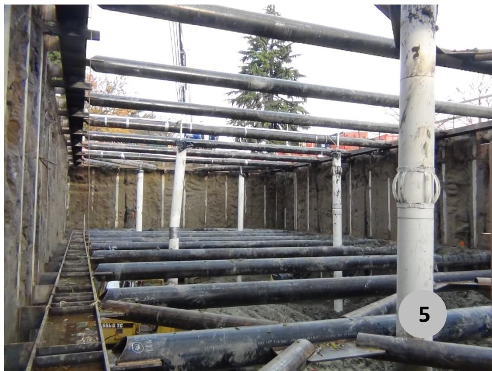
temporarily hold these overflows and prevent them from entering Lake Washington. In order for the reservoir to be constructed CJA was hired to install 278 each 3 foot diameter secant piles with depths of up to 50 feet using the Soilmec 825 and install sheet piling, with 148 tons of internal bracing. CJA's scope of work also included installing 21 dewatering wells.
