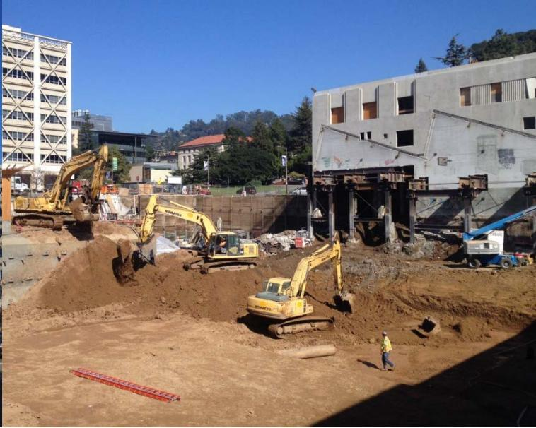
underneath. The temporary steel support structure required over 400,000 lbs of steel with shop drawings, field fabrication, and building jacking all performed by CJA forces. CJA also installed 7,600 SF of soil nail walls, 8,400 SF of soldier pile & tieback walls, and underpinning pits under and around the existing structure.
