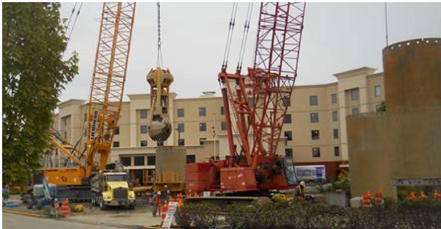
Beginning July 8<sup>th</sup> 2013, CJA began work for PCL installing 70 each 2-meter, 2.5-meter, and 3-meter oscillated drilled shafts up to 170 feet deep for the elevated Southlink light rail extension. When completed, the light rail will be extended by 1.6 miles from Sea-Tac Airport to the new Angle Lake Station on South 200th Street.
