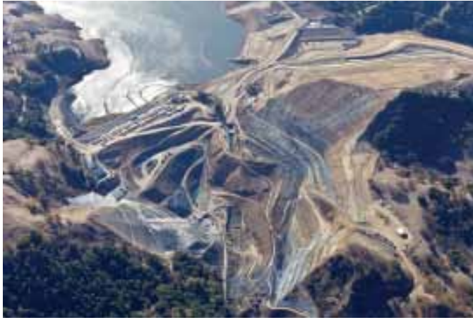
Figure 6. Aerial view of left abutment.
