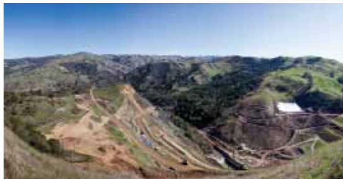
Figure 4. View from left abutment.
