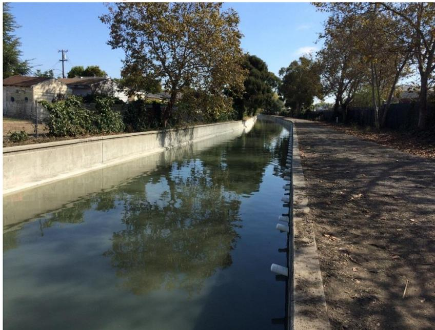
The Corps conducted a preliminary technical assessment in January 2008, and determined that tidal salt water had seeped through the concrete joints and caused severe corrosion of the steel reinforcement near the bottom of this 30-foot section of channel wall. In July 2009 the failed wall section was repaired.
