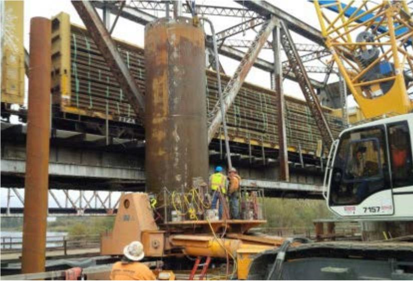
After 106 years of service, the mainline Union Pacific Railroad bridge across the Willamette River at Harrisburg is being replaced. The current structure is a 908 ft. steel truss bridge. CJA was selected by Hamilton Construction to install 18 each 2.2-meter diameter drilled shafts up to 140 feet deep using the 3-meter Leffer oscillator. All of the work is being accomplished during live rail traffic and the shafts are being installed off of a trestle.
