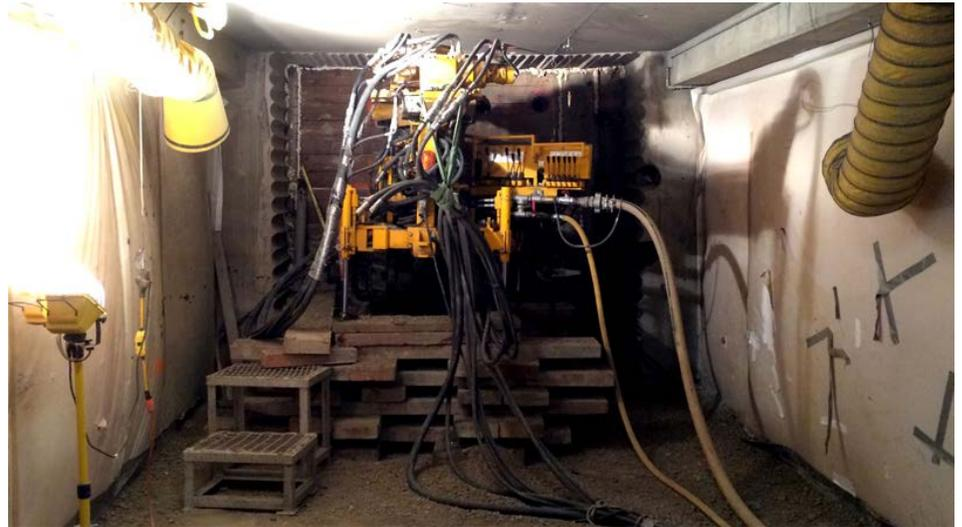
casing (spilling) in a square formation. Each spilling was surveyed with an Inertial Sensing Gyroscope to verify hole alignment before excavation began. The ground is then stabilized via permeation grouting using microfine grout injected through the ports in the casing. The project is being constructed in 3-phases due to the zig-zag pattern of the tunnel.
