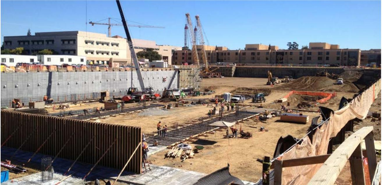
The shoring for the new Adult Hospital and Garage will be complete next month, finishing the Oakland districts' largest and most complex project of the year. In the last 8 months CJA crews installed 533 piles and 924 tiebacks under strict OSHPD inspection. During tieback installation up to 4 Klemms and the Davey-Kent drill were working to meet the demanding project schedule.
