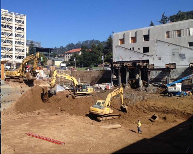
underneath. The temporary steel support structure required over 400,000 lbs of steel with shop drawings, field fabrication, and building jacking all performed by CJA forces. CJA also installed 7,600 SF of soil nail walls, 8,400 SF of soldier pile & tieback walls, and underpinning pits under and around the existing structure.
