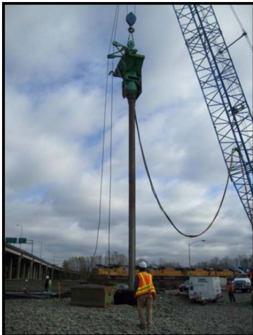
Figure 4. Equipment set-up showing crane mounted vibro-probe
