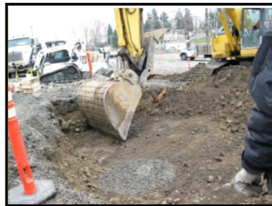
Figure 7. Exposing the top of test section columns
