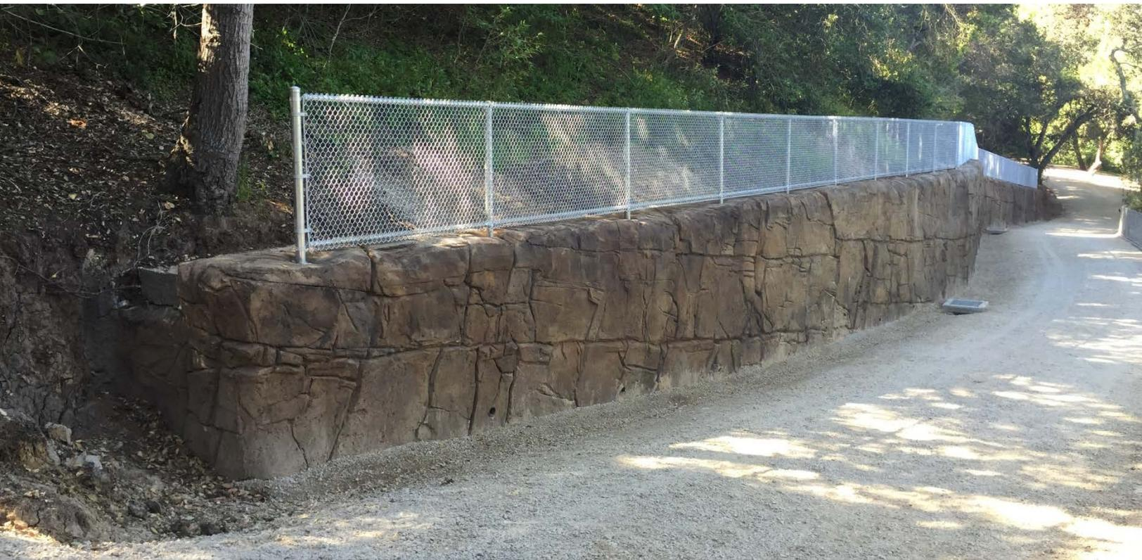
Redwood City contracted with CJA for the construction of a 2,580-square foot sculpted shotcrete retaining wall. In addition to the wall, the project consisted of various site improvements, including road work, installation of a gutter, and general drainage improvements. The purpose of the project was to prevent the existing slope from further erosion while widening the road.
